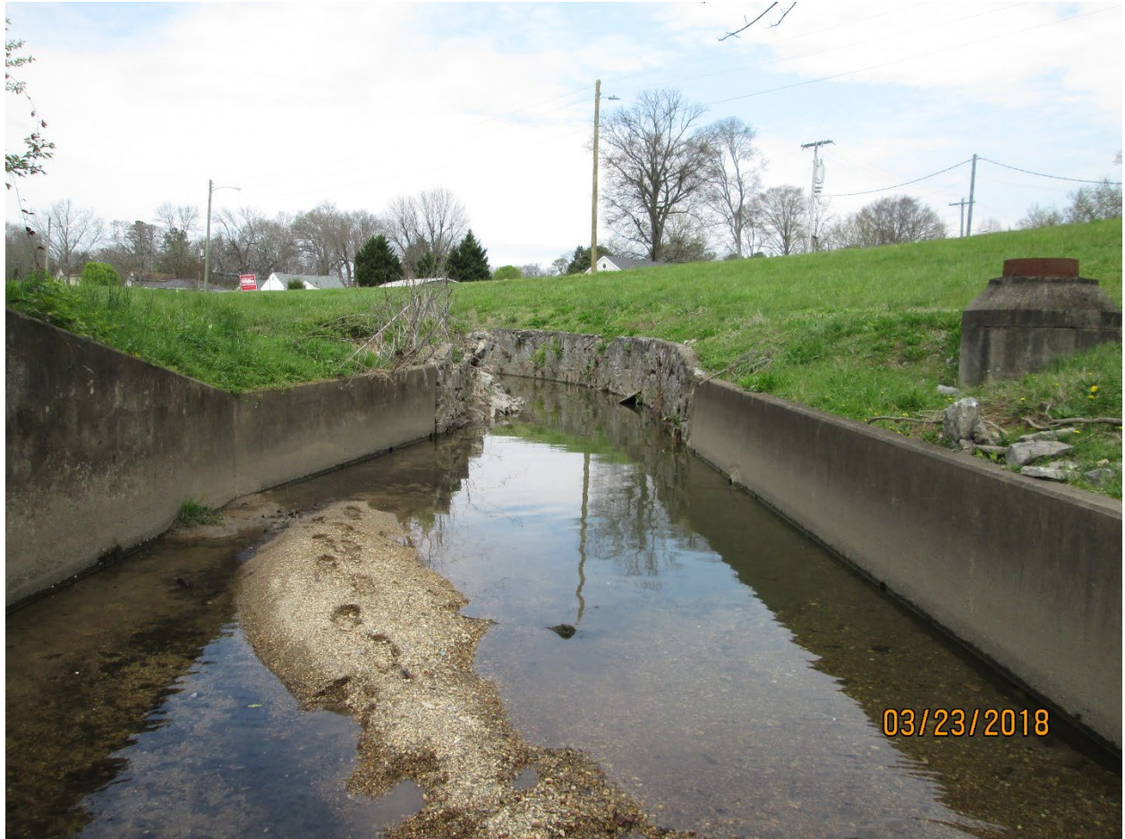
Looking Upstream From I-24/McBrien Road Box Culvert)
