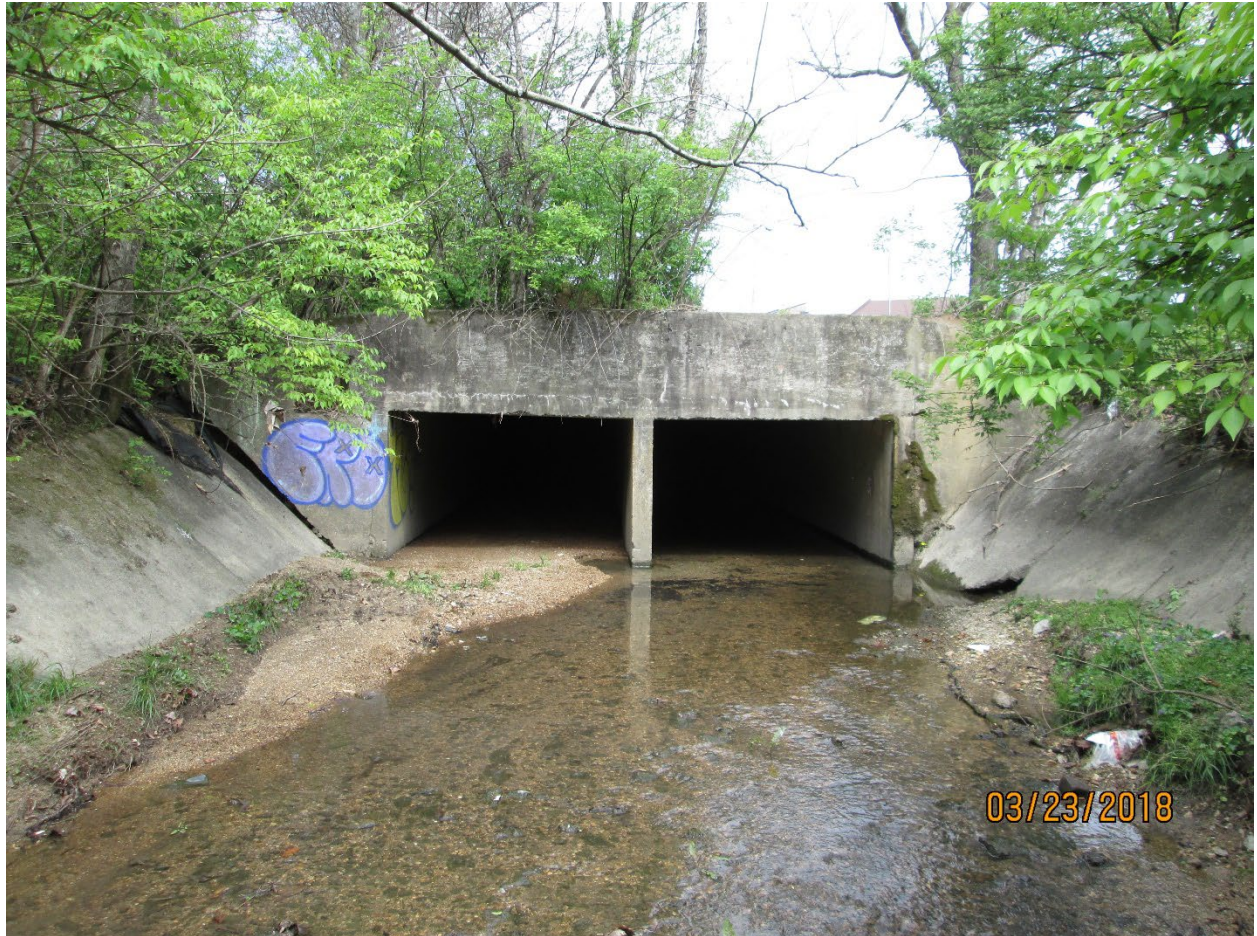
Downstream Face of I-24/McBrien Road Box Culvert)
