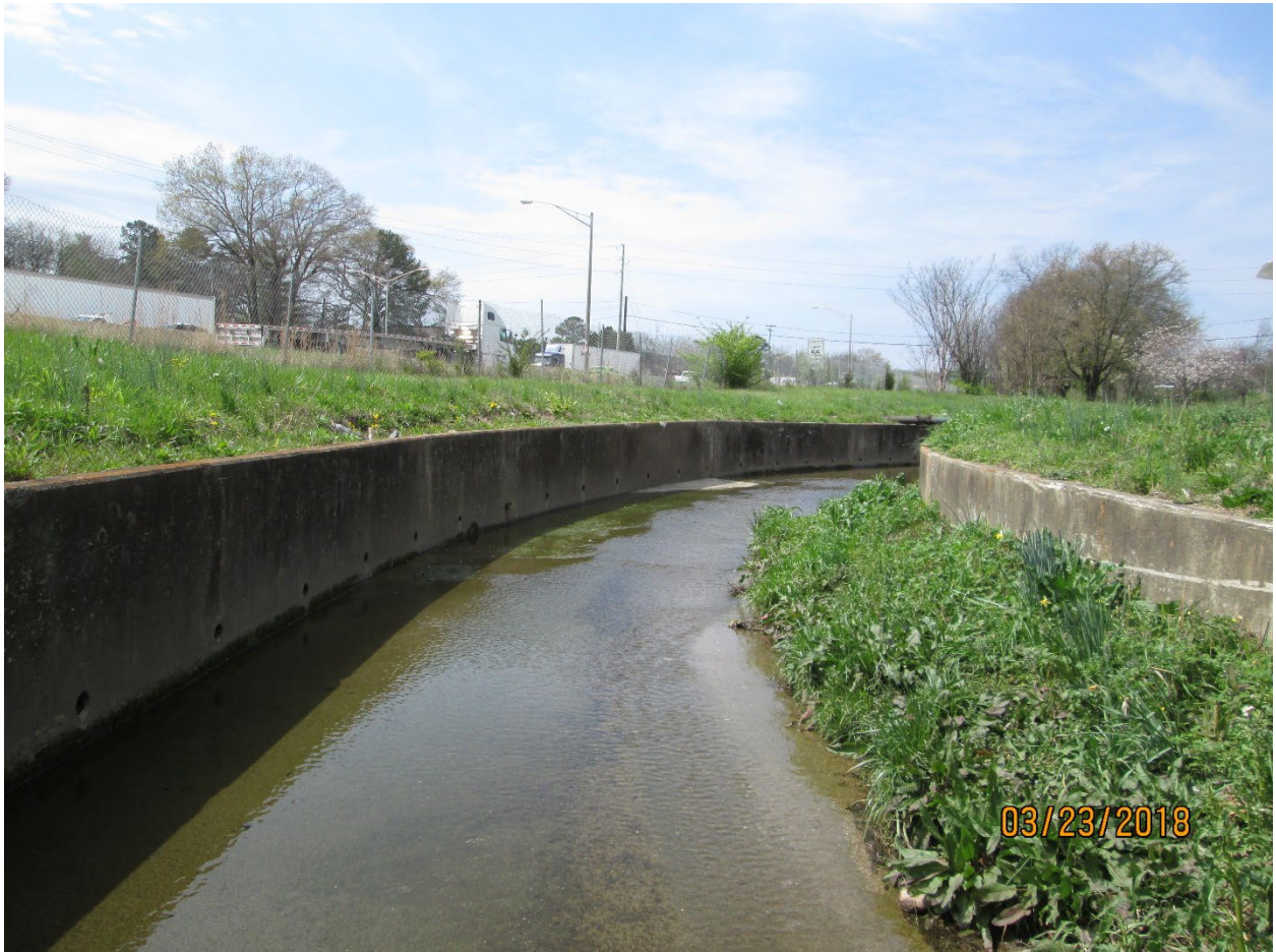
Looking Upstream From Ramp 'O' Box Culvert
