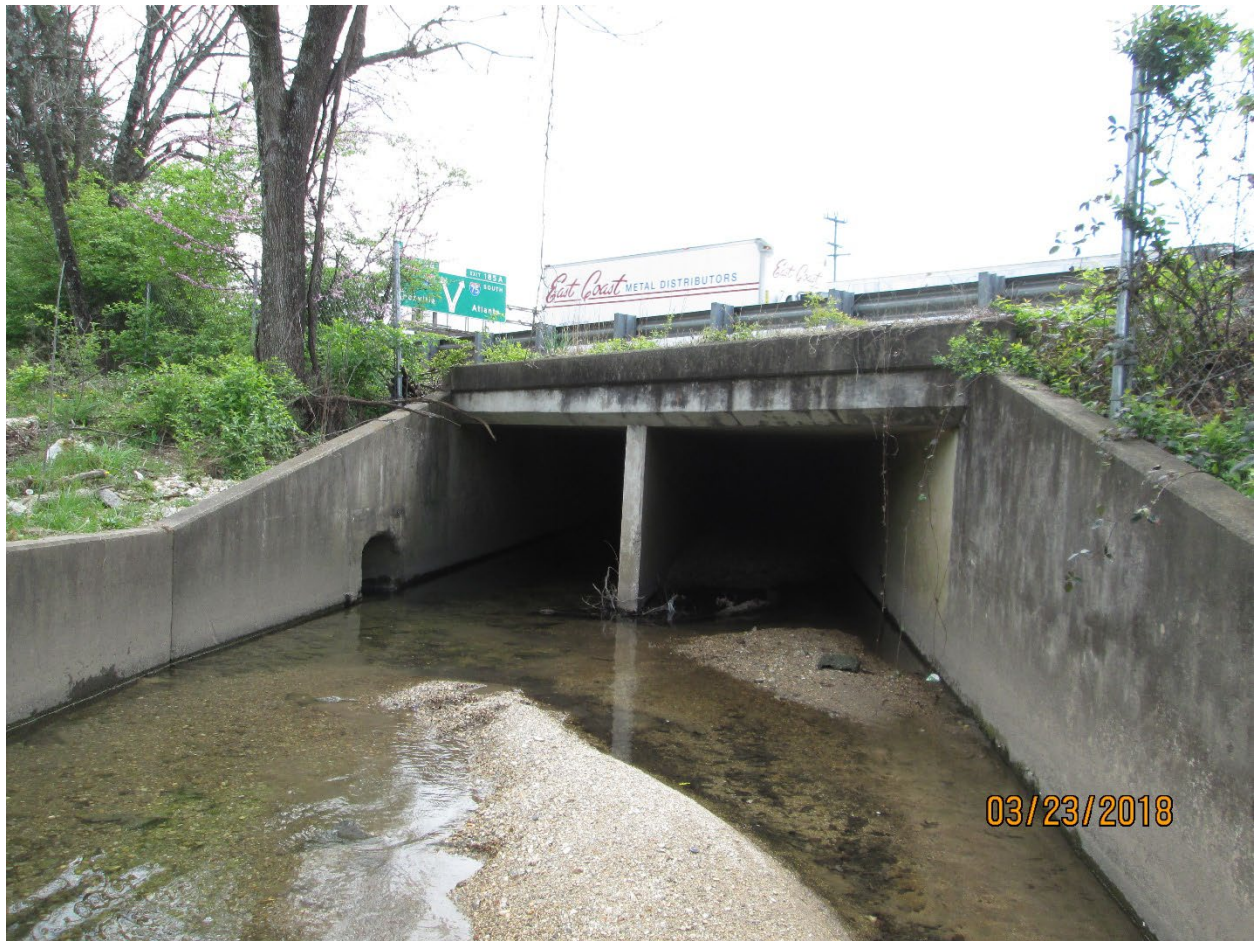
Upstream Face of I-24/McBrien Road Box Culvert)
