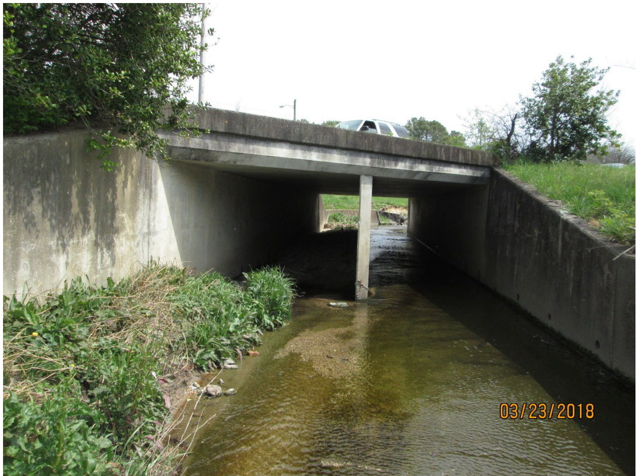
Upstream Face of Ramp 'O' Box Culvert
