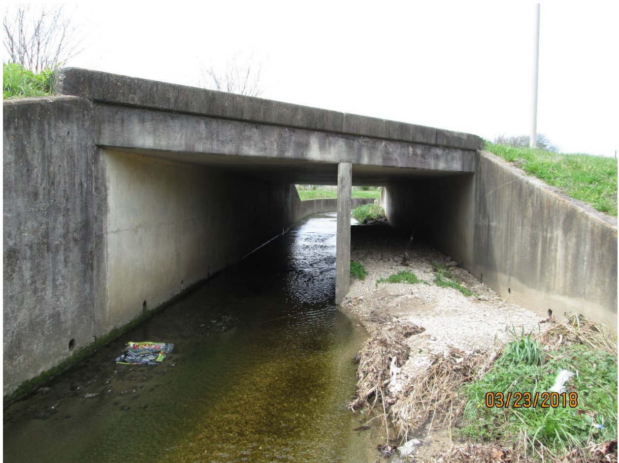
Downstream Face of Ramp 'O' Box Culvert
