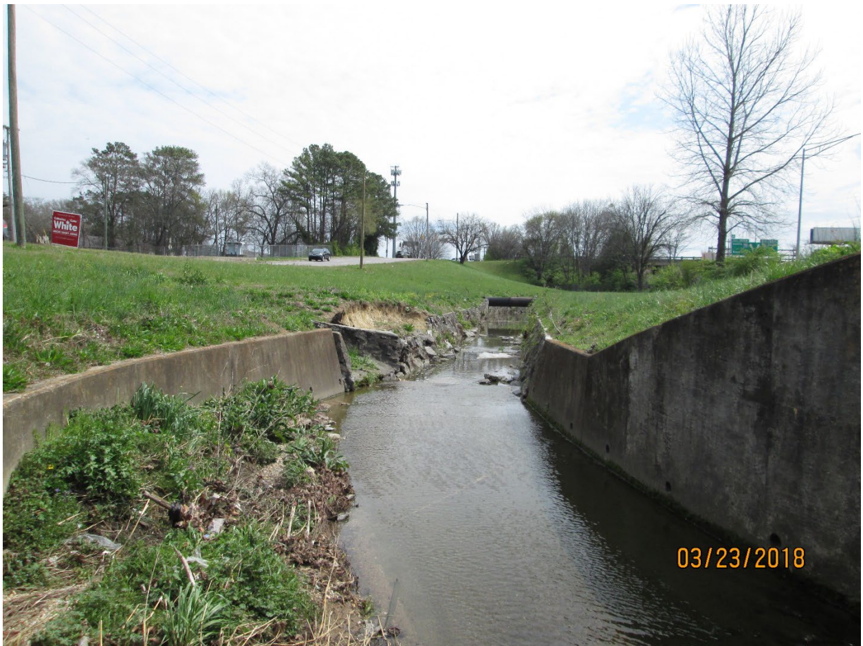
Looking Downstream From Ramp 'O' Box Culvert
